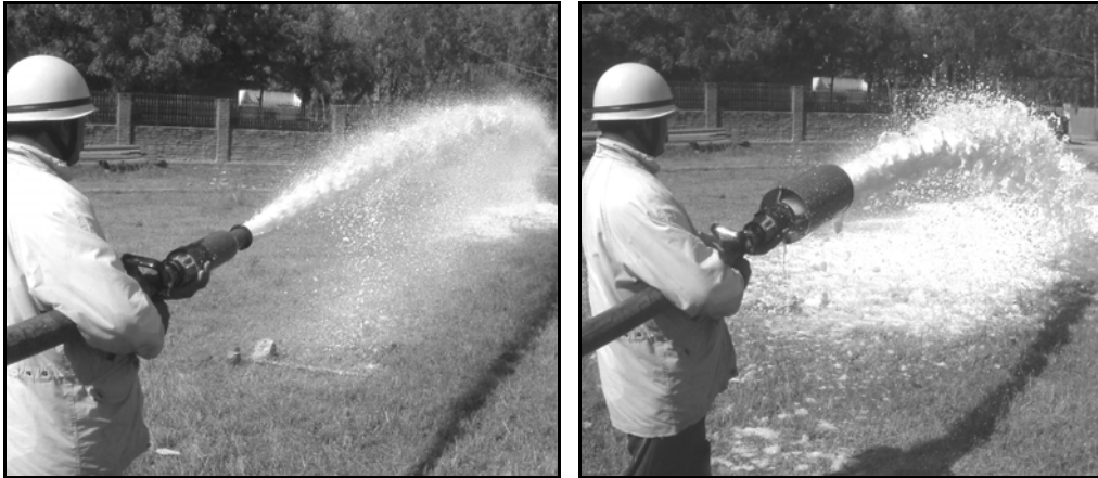
Some nozzles can be used with foam attachments for foam operation. Foam compound can be inducted using Inline Inductors or directly from Foam Tenders.
